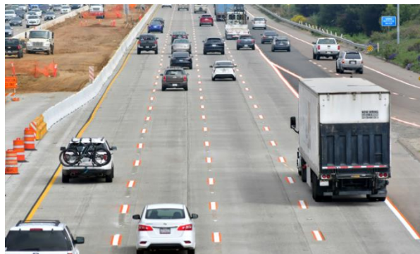
Figure 3. Orange Marking Application on Interstate 5 Northbound
