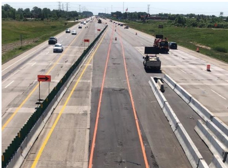
Figure 4. Lane Shift Pavement Markings on Interstate 96
