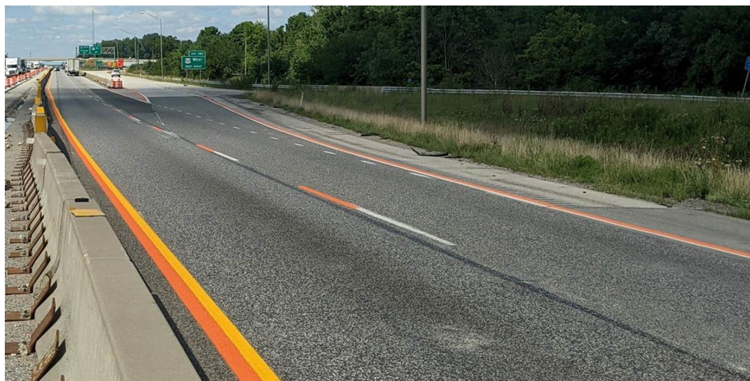
Figure 6. Supplemental Orange Markings on Interstate 65 Northbound
