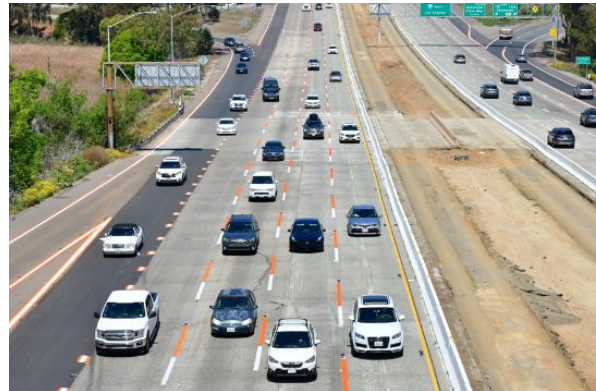
Figure 2. Orange Marking Application on Interstate 5 Southbound
