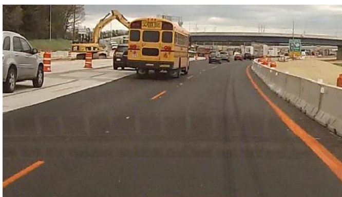
Figure 5. Orange Temporary Marking on Asphalt Surface
