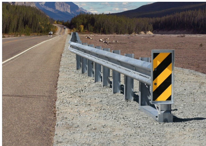
Figure 5. 4F-T™ (4 Foot Flared Trend® Terminal) installed
