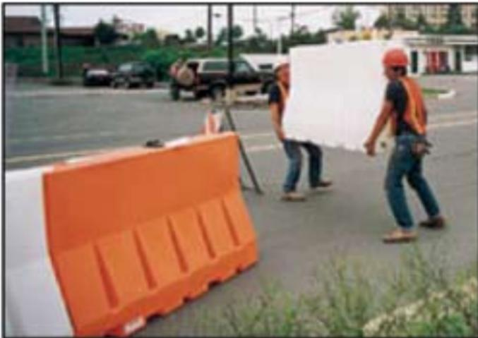
**Figure 3. Empty Ballast-Filled Barrier Segments**
