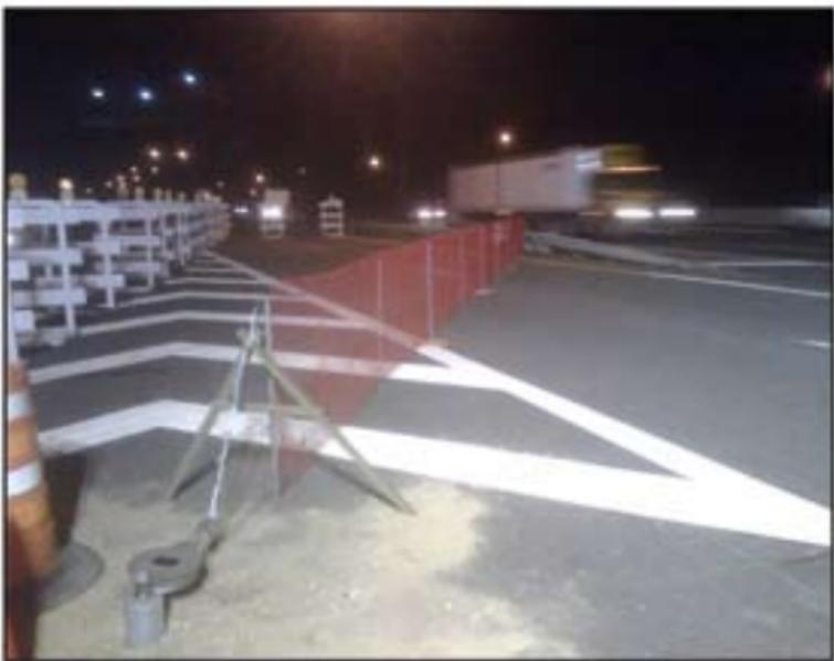
Figure 5. Vehicle Arresting System Protecting Closed Highway Section
