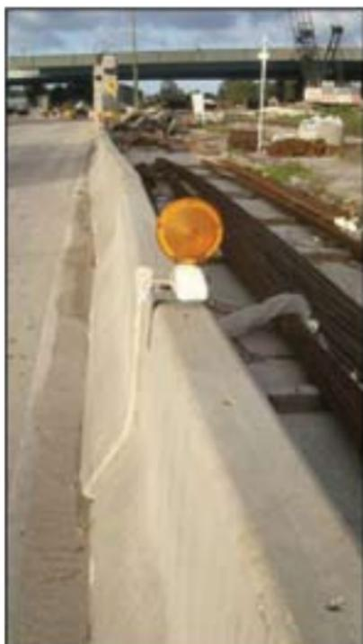
**Figure 1. Portable Concrete Barrier Separating the Traffic Space and Work Space**
